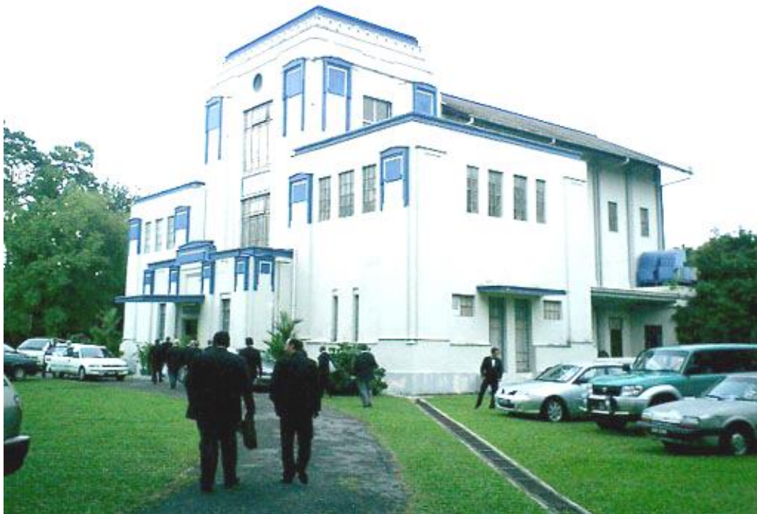
Freemasons Hall, Penang
